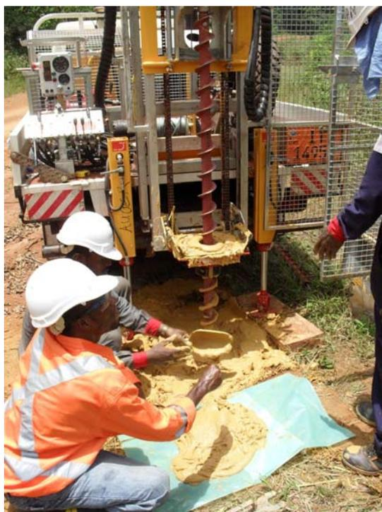
Figure 8: Auger drilling along the Rail Route
